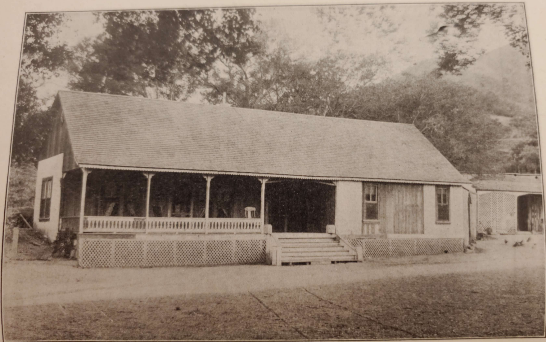
Under the Great Oaks in Griffith Park. (Keeper's Residence.)
